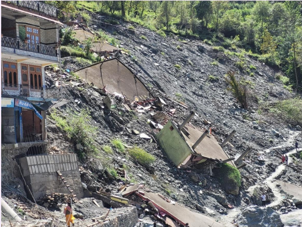
Fig. 2 Devastation due to rainfall-triggered landslides at Sainj area of Kullu district, Himachal Pradesh during monsoon season (2023) - Several houses got washed away blocking the road
