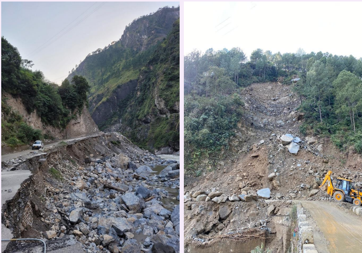
Fig. 1. Swept away sections of National Highway (NH-03) due to flash floods from cloudbursts in Kullu district, Himachal Pradesh (2023) and Landslides in Mandi damaged the under-construction bridge in Mandi district
